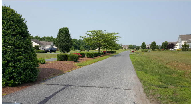
1-1/2" overlay over existing pavement.
